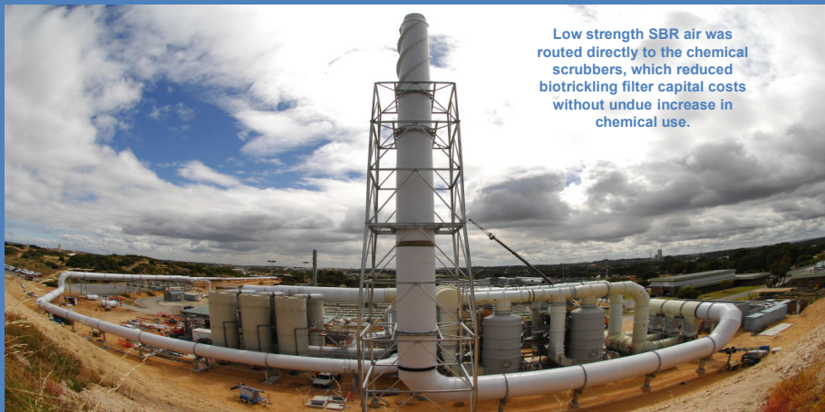
Biotrickling Filter/Chemical Scrubber Odour Control Works at Woodman Point WWTP
