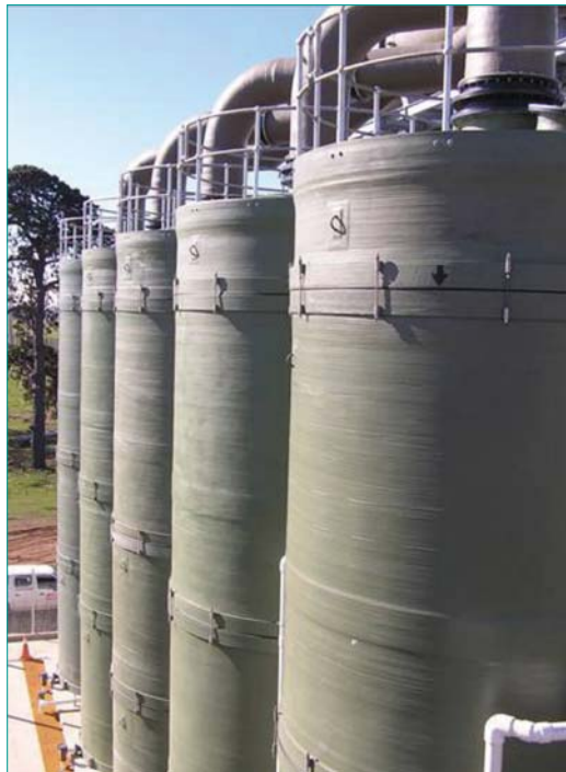
A multi-layered biological odour treatment installation treating 126,000 m 3 /h of odorous air (Cesca et al , 2009).
