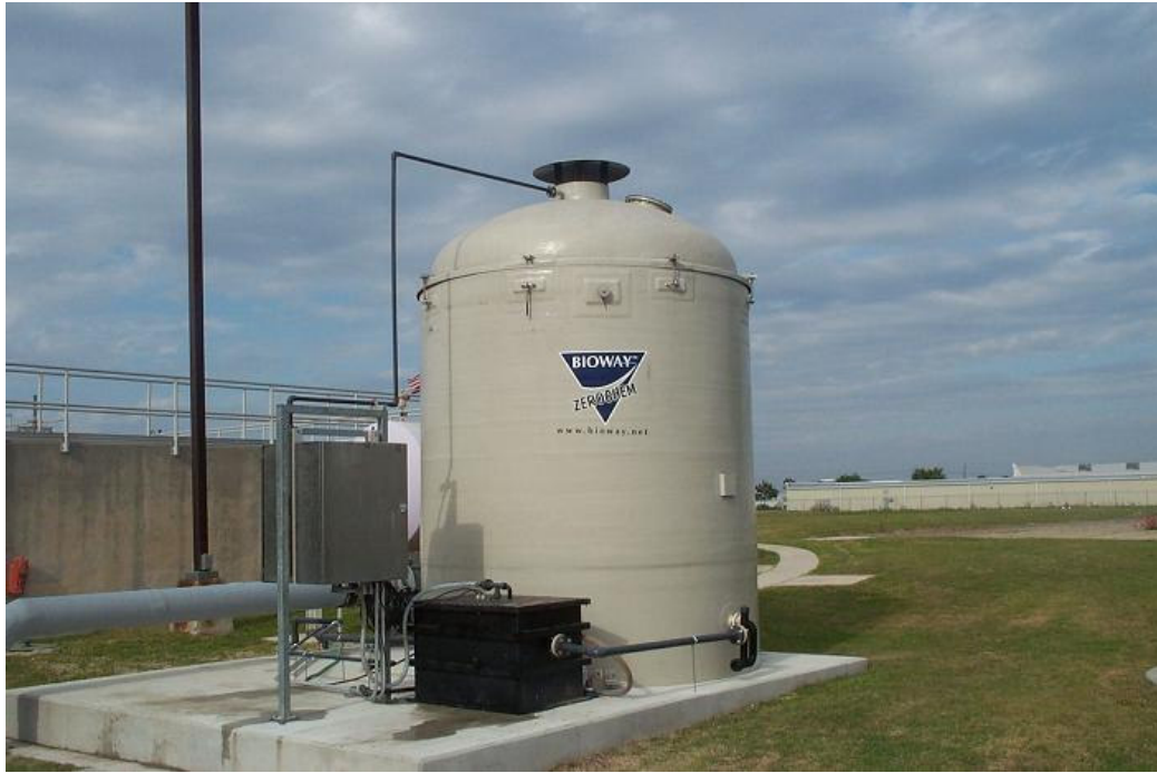
Figure: Biotrickling reactor treating odorous air from at a municipal wastewater treatment plant.
