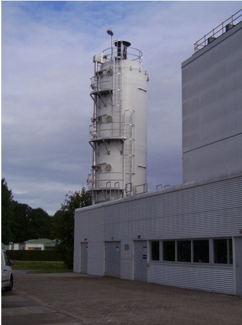
Figure 2: Biotrickling bioreactor treating odorous air from an anaerobic wastewater treatment plant.
