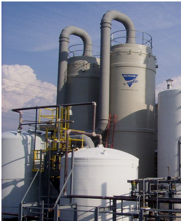
Figure 4: Bioreactors treating CS 2 from waste gas at a fungicide production plant.
