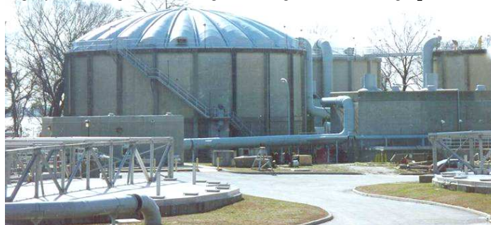
Fig. 5: A municipal wastewater treatment plant.
